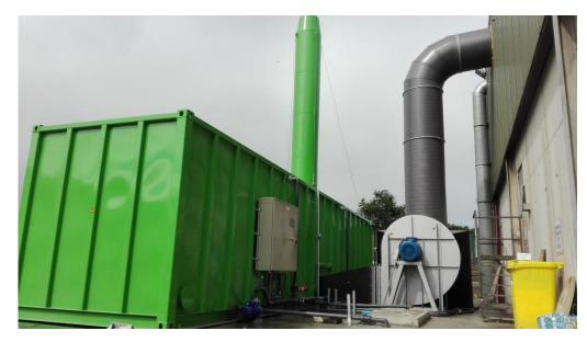
The system is custom made, based on the size of the process hall and the odour load. It can be provided in 1 container processing a flow up to 70 000 m<sup>3</sup>/hour. Depending on the requirements, it can be highly automated and provided with SCADA or other controls which make the system easy to operate.
