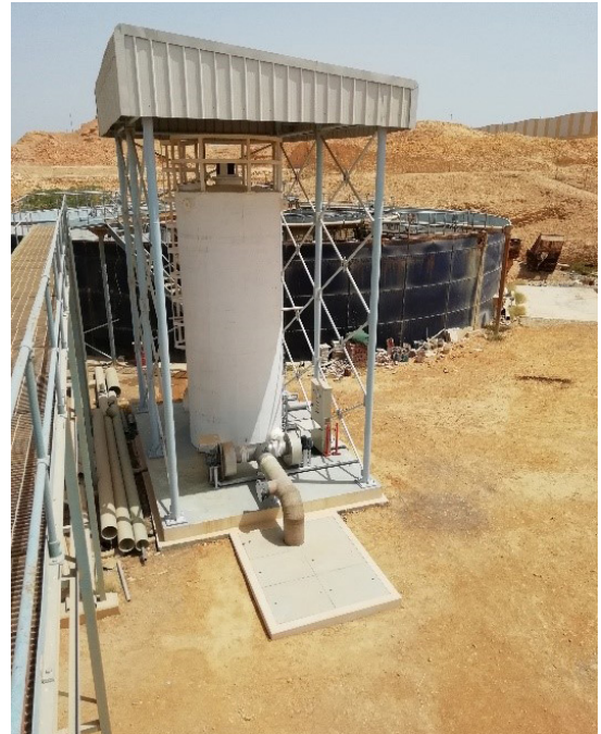
Biotrickling system at Rusayl Industrial Estate (Oman)
