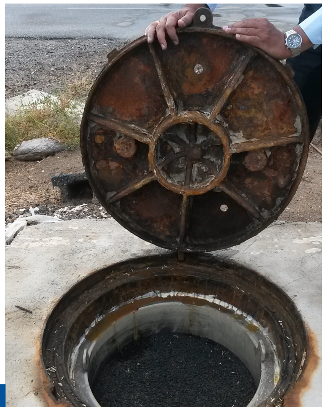
Replacement of damaged seal plate by manhole bucket >
