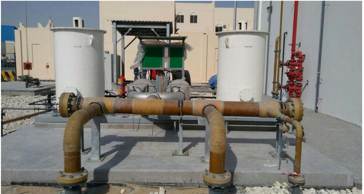
IPEC can supply all kind of activated carbon systems, starting from very small units with the fan mounted on top up to installations with high flows (75 000 m<sup>3</sup>/hour) in vertical or horizontal bed with full automated regeneration, skada connections, etc.
