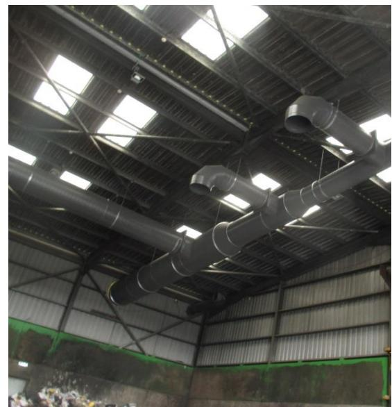
Ventilating the process facility can have some additional benefits for the plant itself since it will improve the indoor climate. The humidity in the hall will be controlled and the corrosion due to the combination of moist with abrasive gasses will be reduced.
